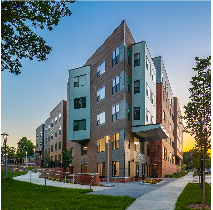
NORTH ELEVATION SHOWING MAIN ENTRANCE, LOBBY AND PEDESTRIAN MEWS ALONG FILMORE AVENUE
