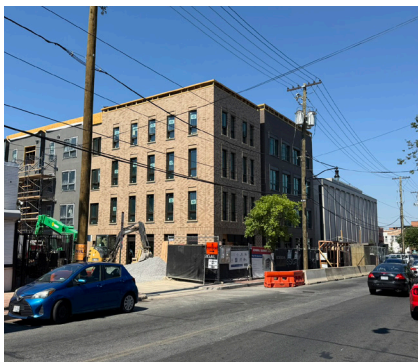
RECENT PHOTOS OF CONSTRUCTION PROGRESS
