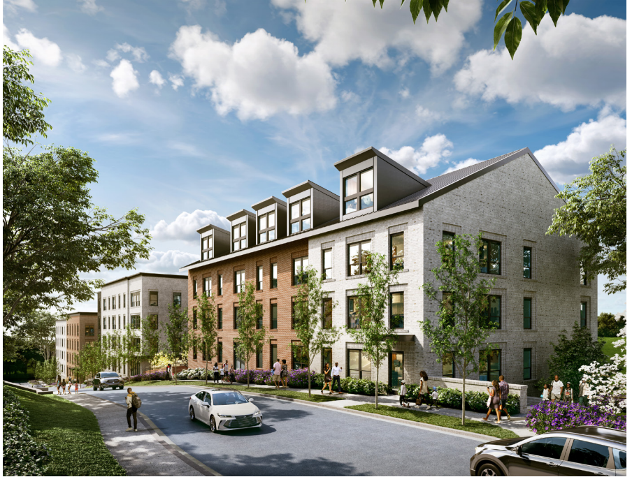
EAST FACADE - NORTH BUILDING
