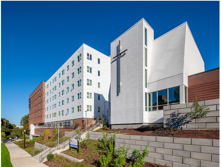
AFFORDABLE HOUSING AND CHURCH
