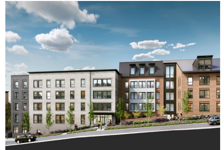
EAST FACADE - NORTH BUILDING
