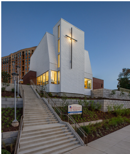
GRAND STAIR AT CHURCH
