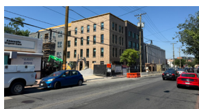
GOOD HOPE ROAD AFFORDABLE MULTI-FAMILY MIXED-USE WITH NON-PROFIT REHABILITATION CENTER (UNDER CONSTRUCTION)
