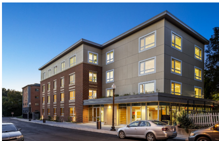
EXTERIOR OF BUILDING
